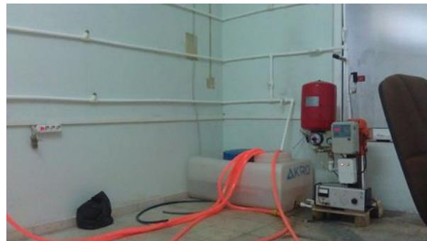
Figure 10 Waterpipeline model of a city deployed wireless pressure sensors
